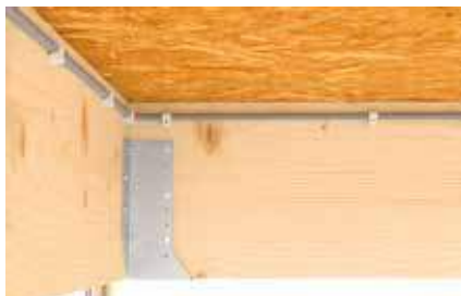
Cable fixing
