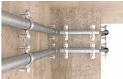
Fixing steel armoured conduits
